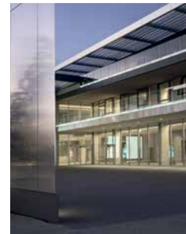
Petronas New R&T Center, workplace, Santena, 2019. Ph. Martiradonna
